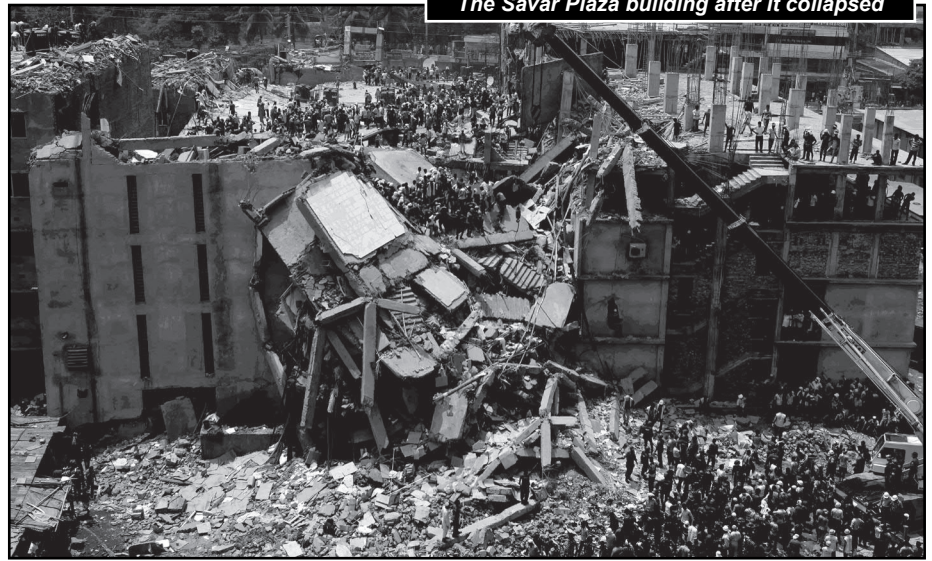
The Savar Plaza building after it collapsed
